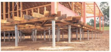
Uni-Piers can be secured to concrete footings with masonry anchors or can be cast into the concrete and allowing the baseplate to become the anchor. Adjustment to the required bearer height is quick and easy by using 14#20 self drilling and tapping metal Tek screws to fasten the head to the post.
