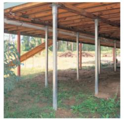
The versatility of Uni-Piers allows a floor system to be easily erected and adjusted to within millimetres on even the most difficult of building sites
