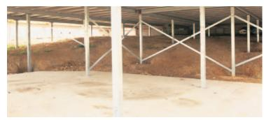
UniPiers will most likely require bracing where the dwelling's walls have cladding. Recommended bracing is 50 x 50 x 2.5mm galvanised steel angle secured with 14#20 self drilling and tapping metal Tek screws. However, bracing may not be required in many situations where the base of the building is constructed with masonry walls.
